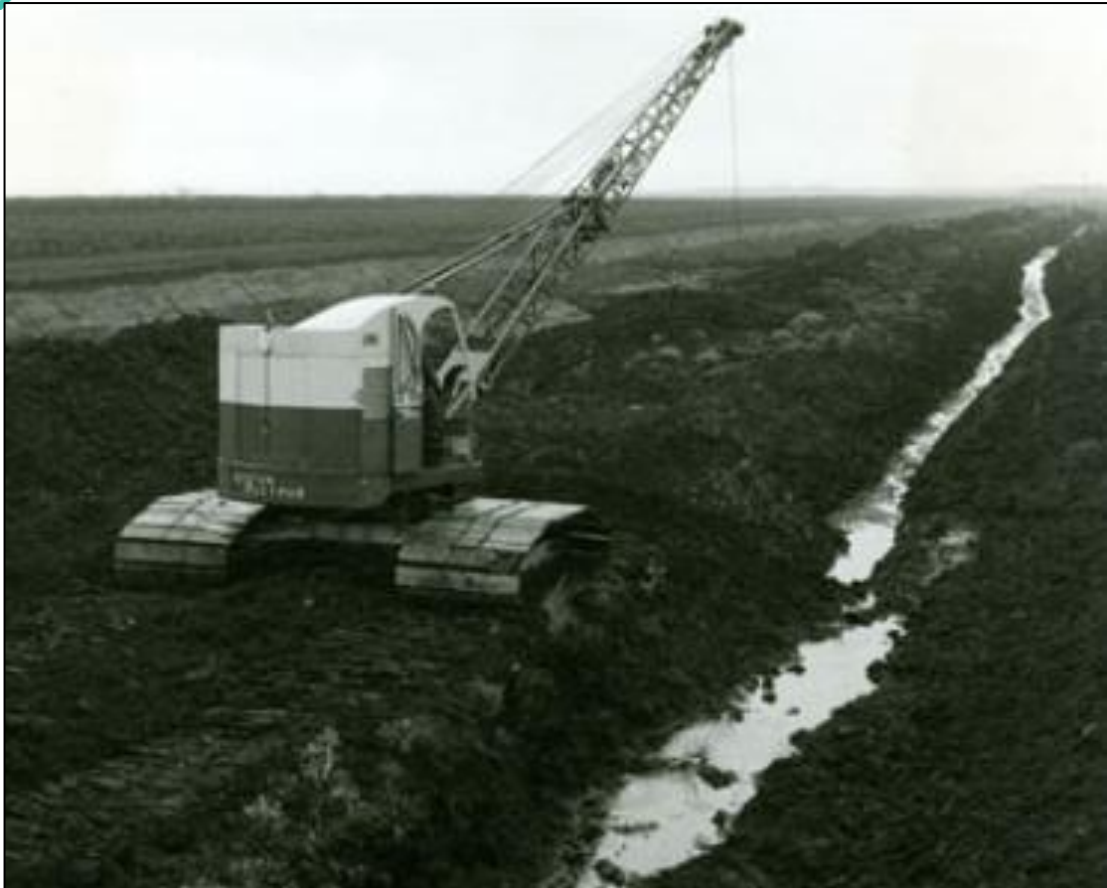
Plate 4- 1 Dragline/Shovel Excavator Source: https://www.bordnaMónalivinghistory.ie/equipment-detail/draglineshovel-excavator/
