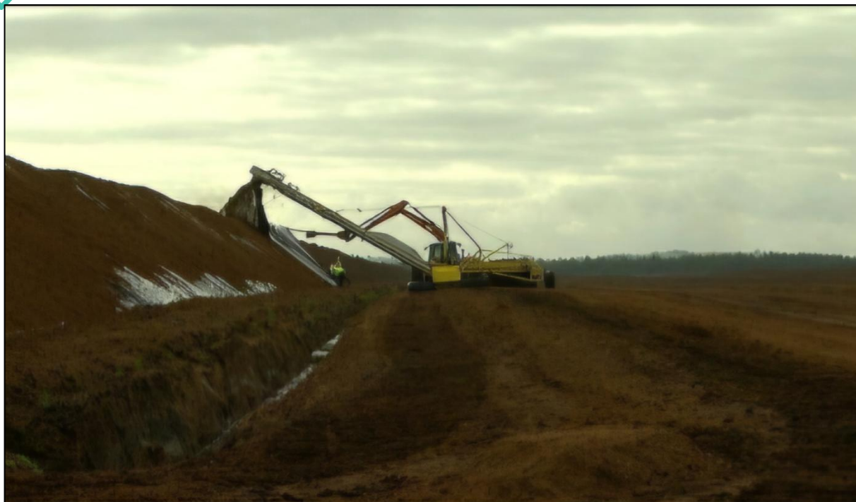
Plate 4- 15 Polythene covering of stockpiles
