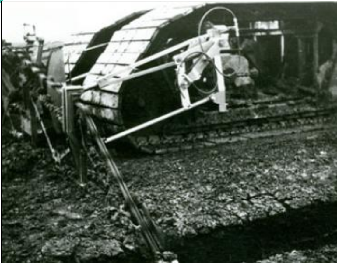
Plate 4-4 Drain Cutting Attachment – Cross Drain. Source: https://www.bordnaMónalivinghistory.ie/equipment-detail/drain-cutting-attachment-cross-drain/
