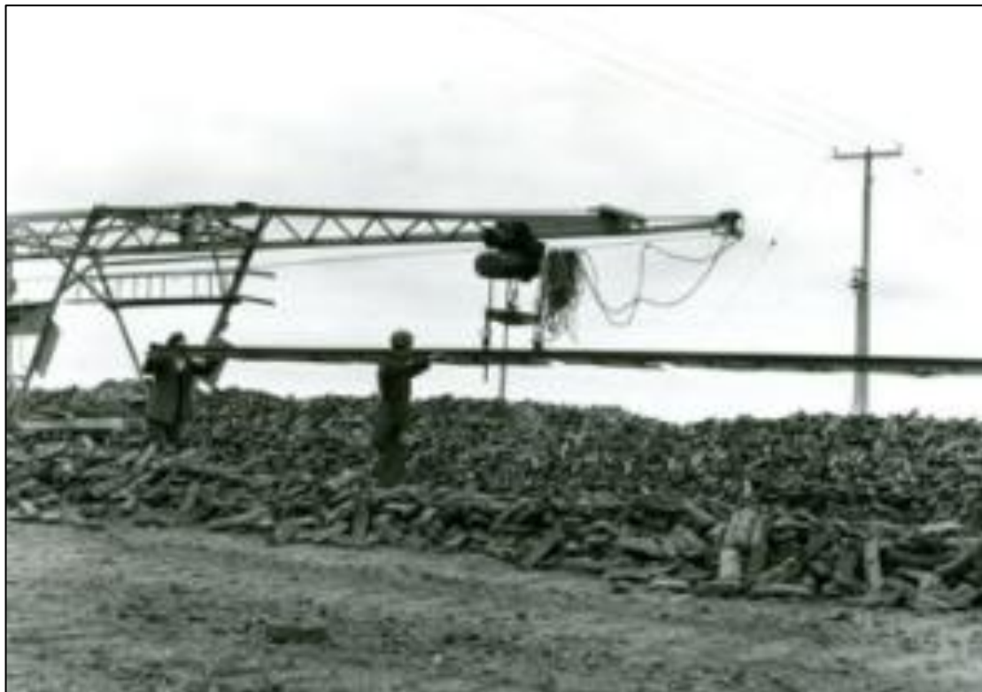
Plate 4-35 Rail Shifter. Source: https://www.bordnaMónalivinghistory.ie/equipment-detail/rail-shifter/
